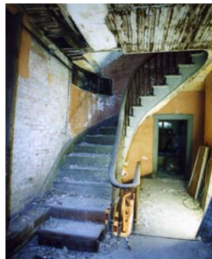
Second floor staircase
