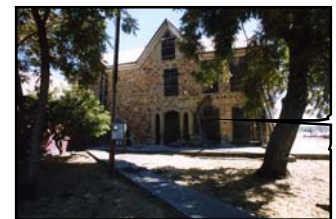
Newly repaired west wall
